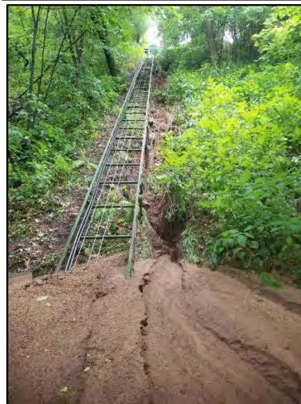
Mud and sediment tracked out into roadway. Sediments tracked out must be swept daily .
