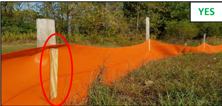
Fence tight, trenched in , secondary piece of lath used for reinforcement.
