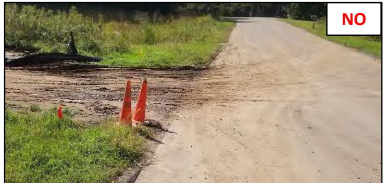
Mud and sediment tracked out into roadway. Sediments tracked out must be swept daily .
